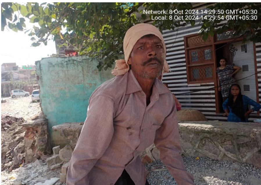
Guhli Talab - New Room Build up old wall removed
