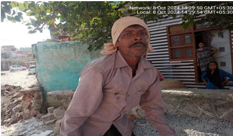
Guhli Talab - New Room Build up old wall removed
